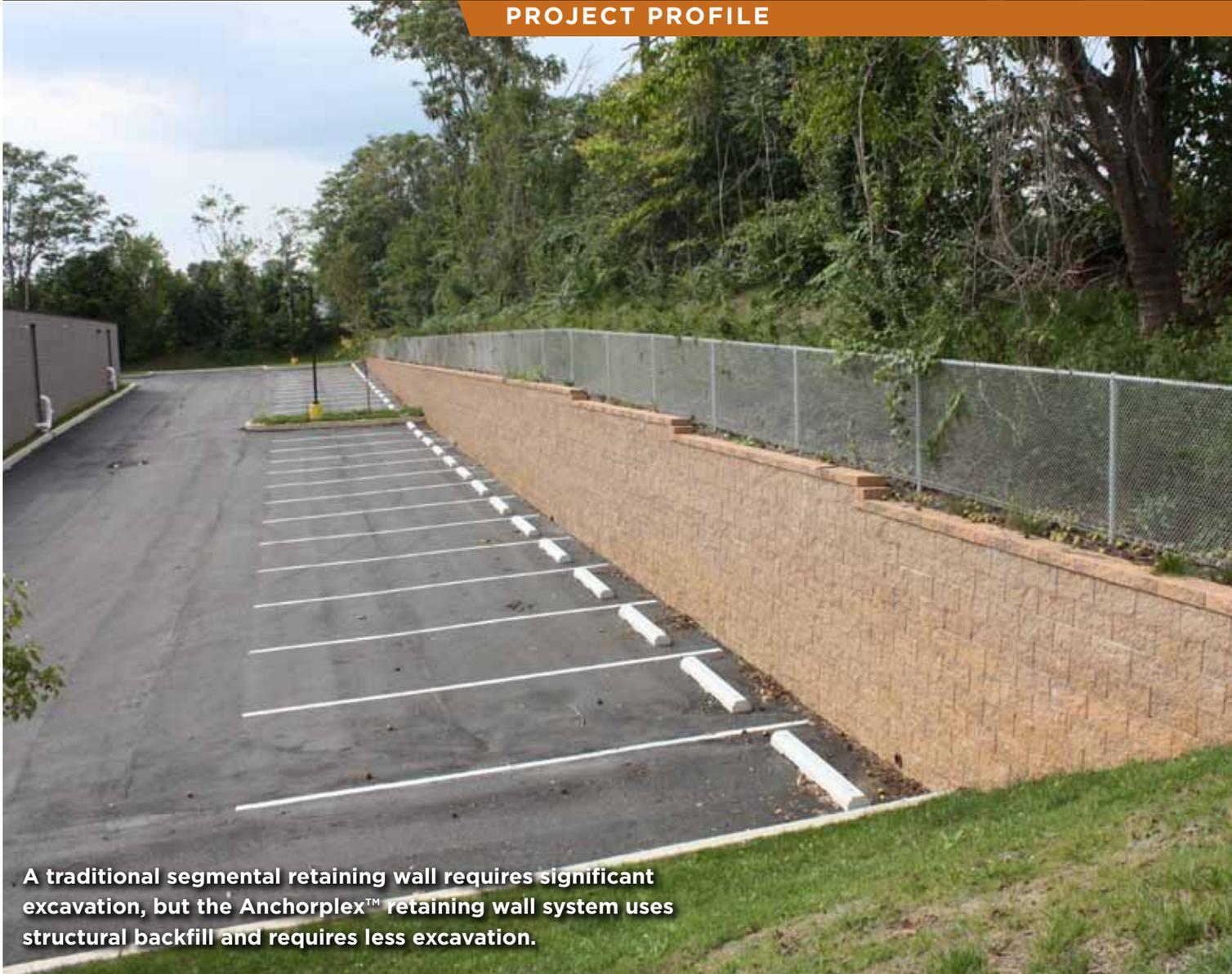
A traditional segmental retaining wall requires significant excavation, but the Anchorplex<sup>™</sup> retaining wall system uses structural backfill and requires less excavation.
