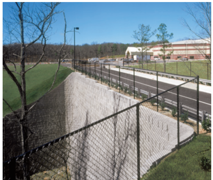
This land bridge provides much needed access to overflow parking.
