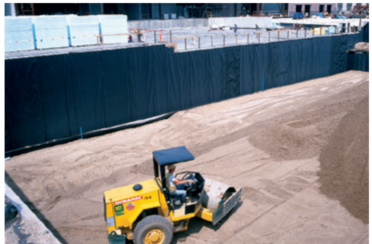
Project site near wall completion.
