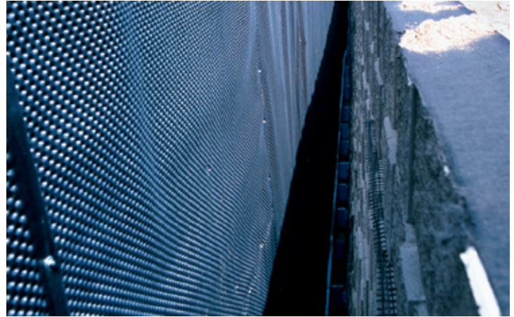
Project site mid-wall construction.
