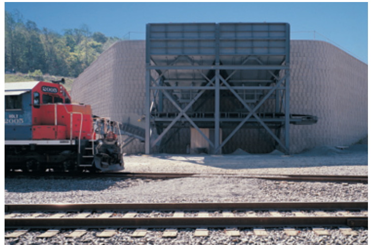
The hopper-loading facility is connected to the high-load-bearing wall with a concrete slab.
