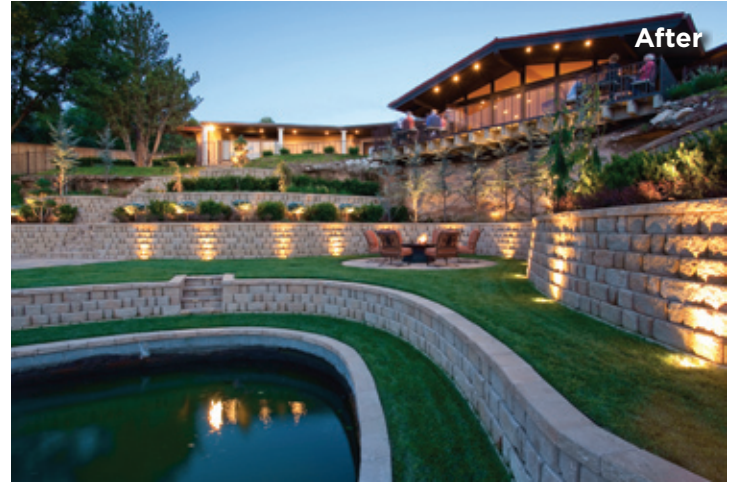
Terraced retaining walls hug the contours of this challenging site and provide safe access and planting areas.
