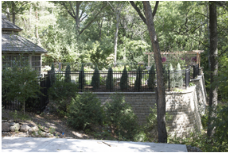
The new backyard is supported by a Highland Stone® retaining wall.
