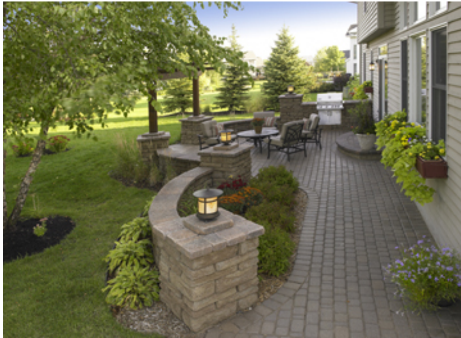
The completed project.
