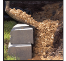
5. Add Drainage Aggregate
