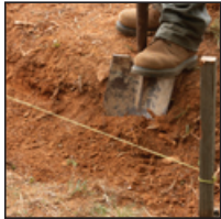
1. Stake Out/Remove Sod
