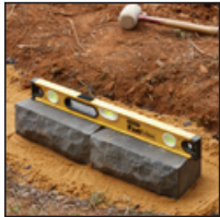
4. Lay and Level Blocks
