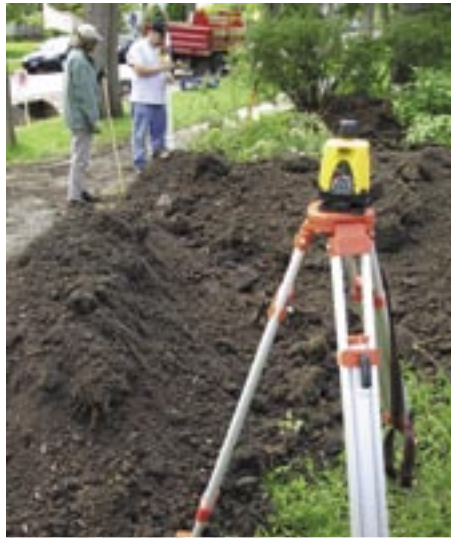
Use a transit and a laser level to calculate wall height.
