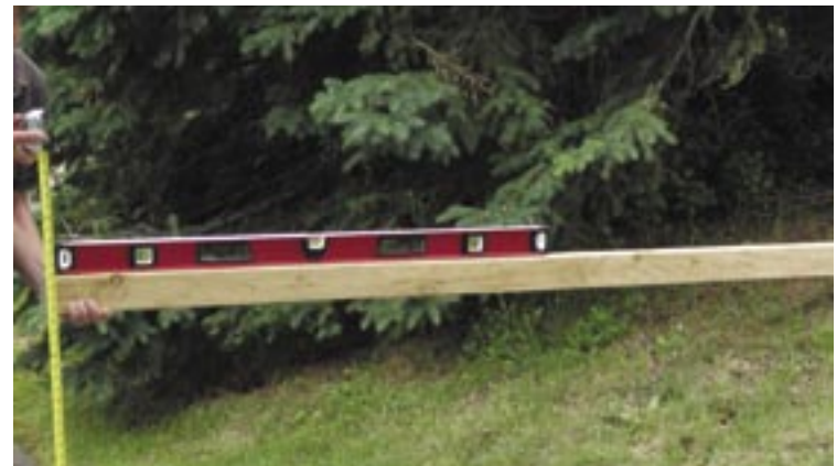
Using a 2x4 and a level to calculate wall height.
