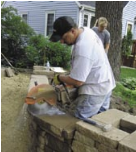
If cap units are not lying neatly next to each other, "butter cut" them until they touch smoothly.
