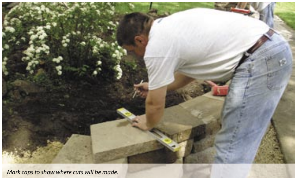
If cap units are not lying neatly next to each other, "butter cut" them until they touch smoothly.
