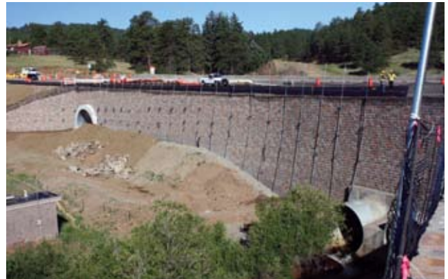
The Shaffer's Crossing interchange included segmental retaining walls that reached heights of 53 feet. To meet the high aesthetic standards of the project, two colors of the Diamond Pro Stone Cut wall system were installed randomly.
