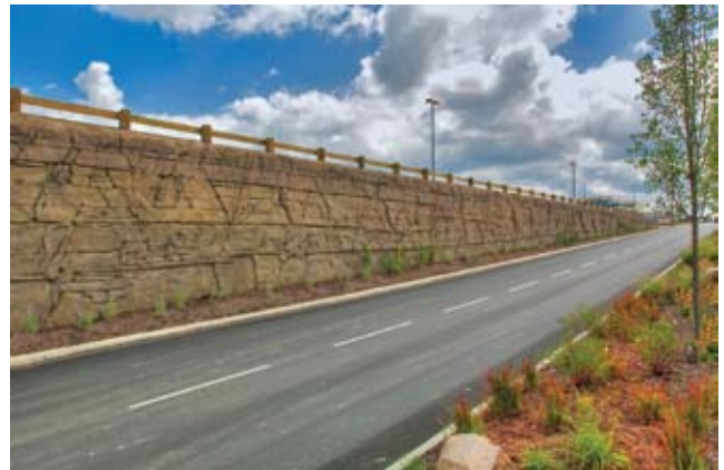
A shopping center developer in Ohio challenged Boulderscape to apply a fractured rock granite finish that matches the area geology to a series of seven retaining walls.
