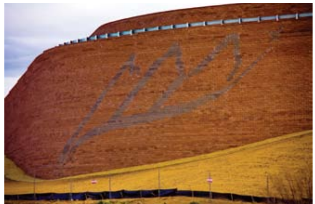
The Rocky Mountain Metropolitan Airport's retaining wall features the airport's logo built out of Compac II segmental units in a contrasting color.
