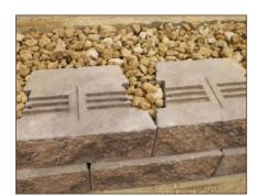
Diagram 8-Backfill and Fill Voids
