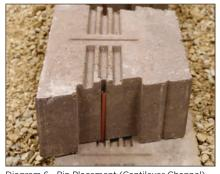
Diagram 6-Pin Placement (Cantilever Channel)
