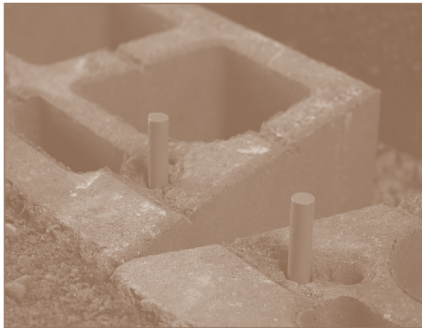
Diagram 5—Pin Placement
