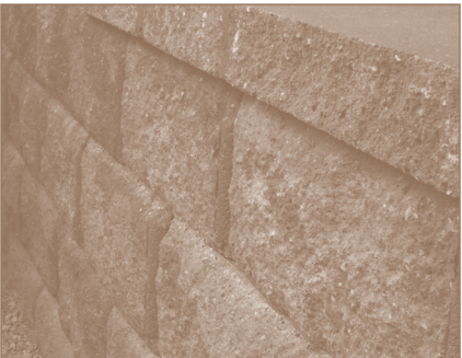
Diagram 10—Capping
