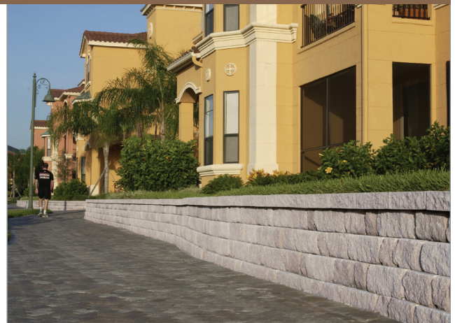
Each parking lot was separated from the landscape by a retaining wall that defined the grade.
