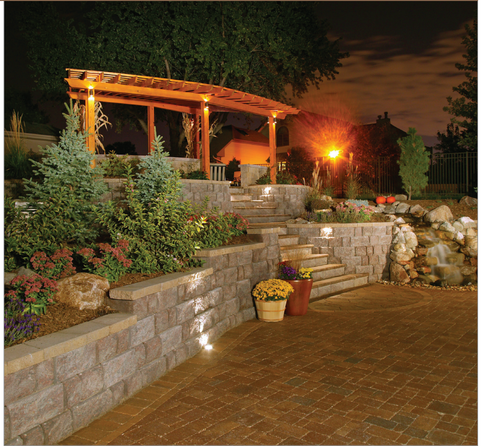
The Diamond Pro Stone Cut® retaining wall system along the pool patio harmonizes with the landscape.
