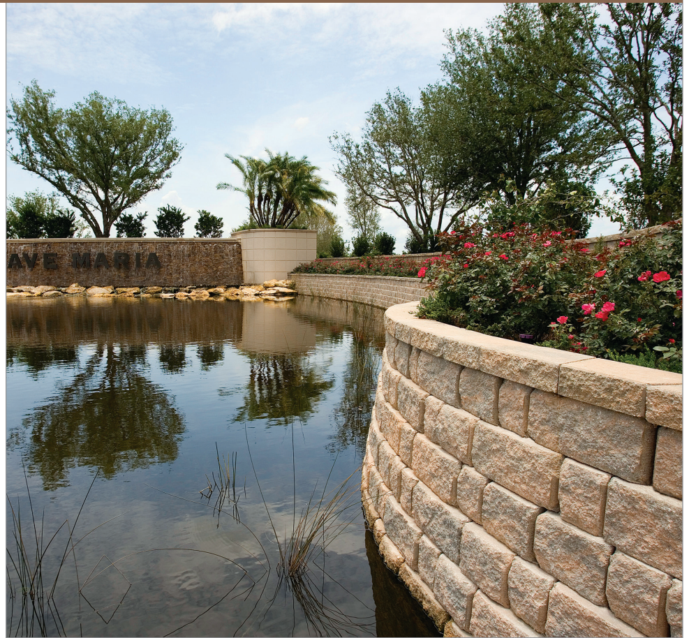
The Diamond Pro Stone Cut® retaining wall system was used to create the entrance sign to the Ave Maria community.
