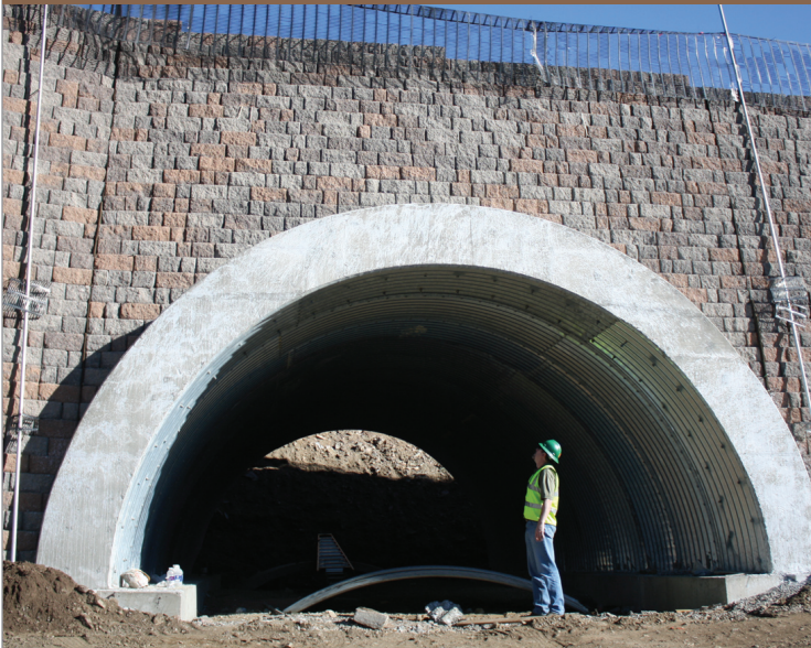
The retaining wall was built to accommodate large culverts for spring flooding and to provide a passage for wildlife.
