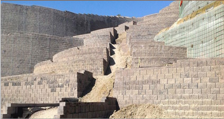
20 planter walls create a stairway to the upper retail pad. Elevation change is approximately 100 feet.
