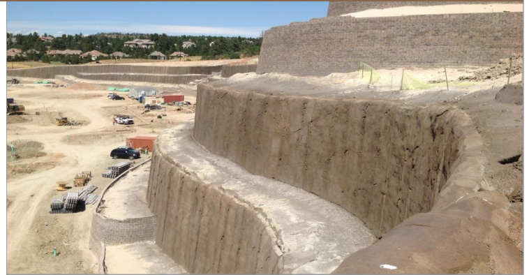
Anchor™ Diamond Pro® wall with sculpted shotcrete facing creates the look of natural rock outcropping.
