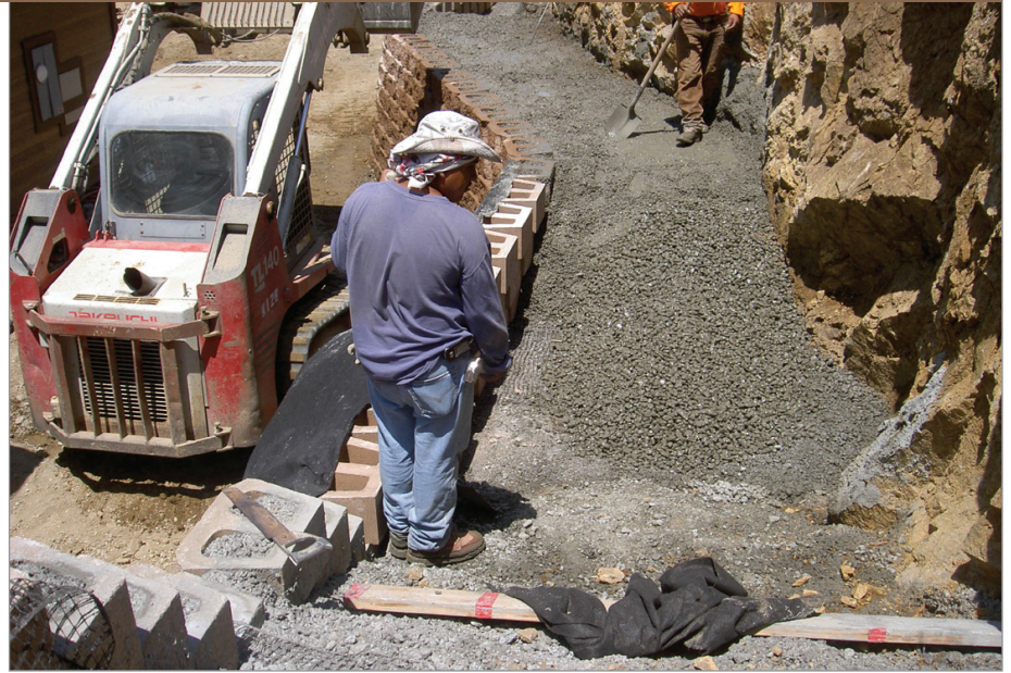
The Anchorplex™ retaining wall system uses segmental retaining wall units, which are backed with a zone of structural backfill.
